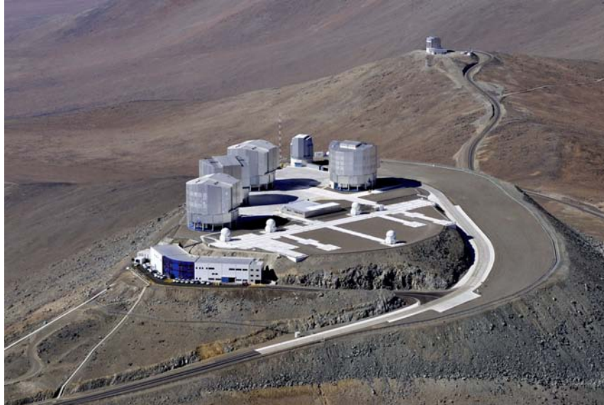
Figure 1. ESO site on Cerro Paranal. The VLTI is formed by four Unit Telescopes with main mirrors of 8.2m diameter (large buildings) and four movable 1.8m diameter Auxiliary Telescopes (domed buildings). Picture by ESO.
